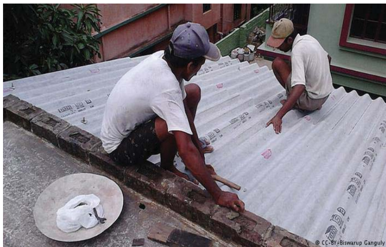
Workers install a roof in India using corrugated asbestos sheets
